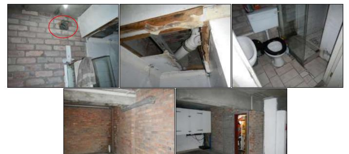
**In pictures 1-4** we see that the forced ventilation servicing the caretaker's bathroom (toilet, hand basin and shower) has been removed, this area must be mechanically ventilated, and the in-line fan and grille must be reinstated.
