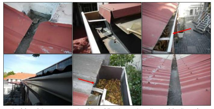
**In pictures 1-6** we see examples of the existing storm water gutters servicing the roof areas of the complex. These gutters generally, appear to be in a good condition, with no major leaks or defects noted during our visual inspection. We do however note that several gutter sections and hopper boxes are blocked with leaf matter and likely to restrict the flow of water. Immediate cleaning is recommended.
