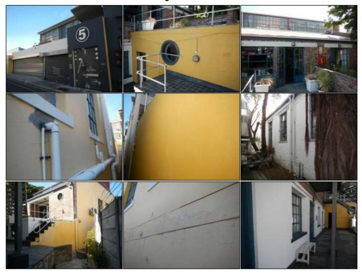
**In pictures 1-9** we see examples of the existing walls, which generally appear to be in a moderate condition, with degradation such as cracking of the plaster and failure of the coating evident in several areas.
