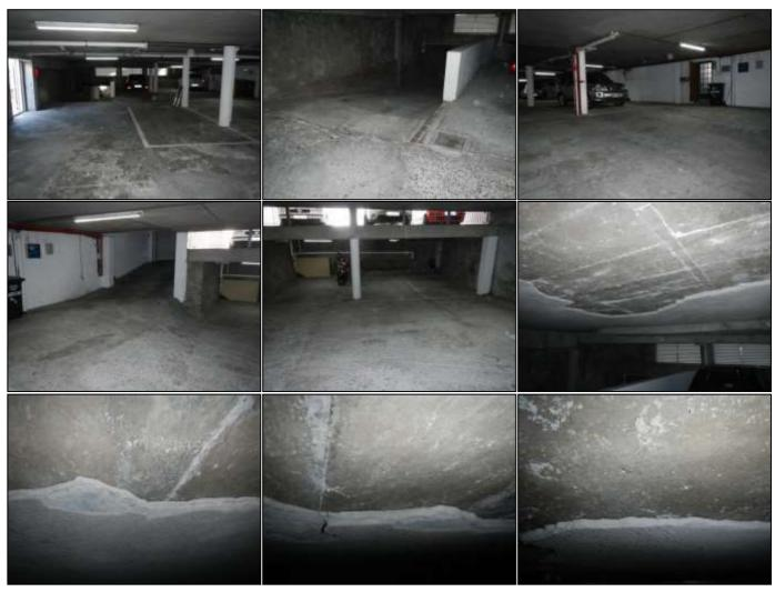
In pictures 1-6 we see an overview of the undercover parking area. The parking walls and soffits areas are generally in a moderate to poor condition with obvious coating failure as a result of general wear and tear as well as water damage.
