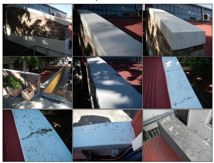
**In pictures 1-9** the masonry tops/parapet wall sections are generally in a moderate to poor condition, with obvious coating/paint failure and cracking evident in areas.
