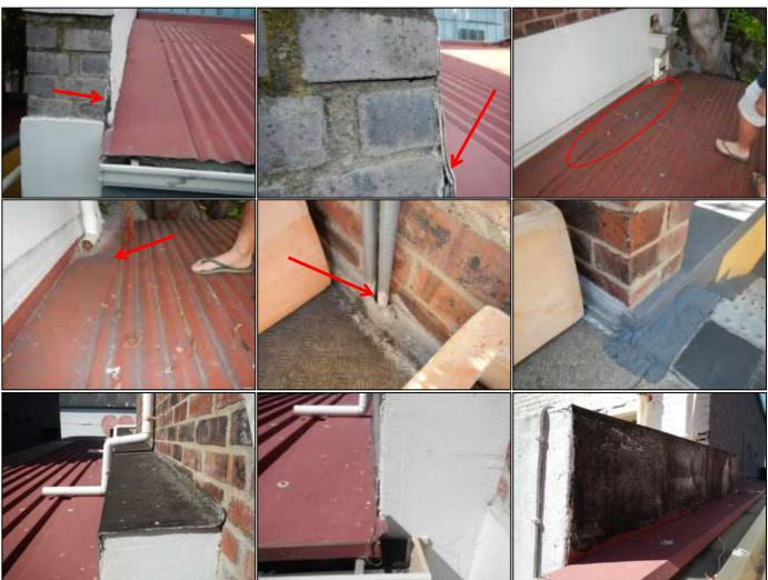
**Pictures 1-9** are examples of existing capping's and flashings which generally appear to be intact however do note some obvious defects in areas.
