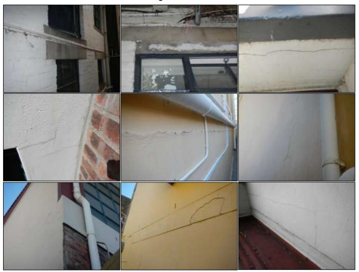
As seen in pictures 1-9 we see examples of cracking and plaster delamination evident to various areas of the exterior of the building complex.
