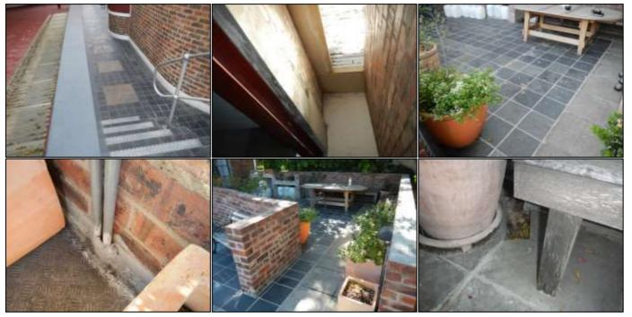
**In pictures 1-7** we see examples of the existing (tile surface finish) flat roof areas. Defects and leaks into unit 18 and common walkway underneath these areas were brought to our attention on the date of our inspection.
