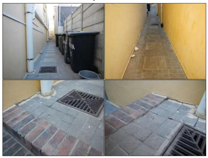
In pictures 1-4 the paved sections/areas generally appear to be in a fair and functional condition and note no widespread degradation or sagging of these surfaces has been noted.
