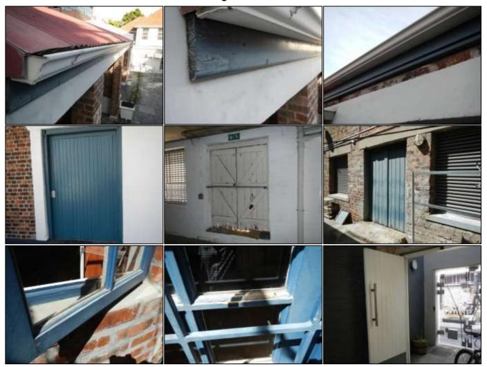
**In pictures 1-9** we see examples of paint woodwork that is generally in a moderate to poor condition, with severe weathering and possible wood rot evident in areas.
