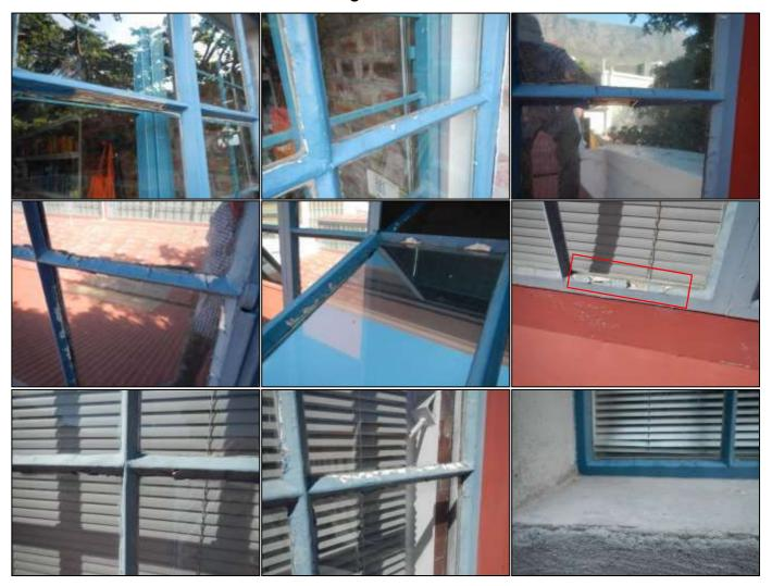
**In pictures 1-9** we see examples of defective putty to the various metal windows within the complex. The window putty was found to be defective to many of the mild steel window units inspected.
