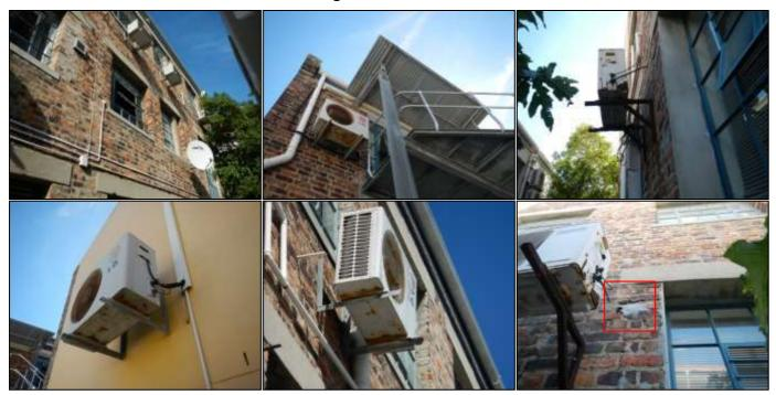
**In pictures 1-4** we see the existing air-conditioning units appear to be in a moderate working order and note rust creep/corrosion of the casing was observed during our visual inspection and requires maintenance. (We assume this is of the owners account to maintain)
