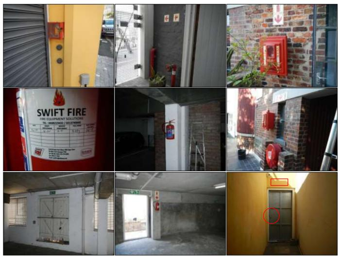
**In pictures 1-9** we see examples of the existing fire equipment and emergency signage. All equipment appears to be in a good working condition and to have been maintained regularly.
