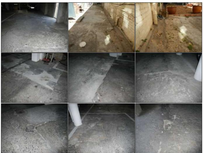
As seen in pictures 1-9 the concrete walkway/service areas are generally in a poor condition, with obvious cracking and defects of the concrete surface visible in many areas.
