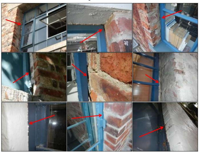
**In pictures 1-9** no evidence of wall to frame seals has been noted in between the wall and window frame.
