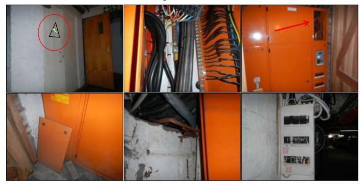
**In picture 1** we note that the electric hazard sign has not been fitted to the access door. This must be implemented to ensure compliancy.
