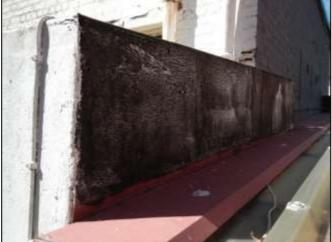
**In pictures 1-3** we see an overview of the exposed waterproofing to the parapet wall areas. These roof areas comprise of a Talc heat fused membrane system (also known as torch on). All sections inspected, appear to be in a moderate to poor condition, with obvious failure of the protective coating evident.
