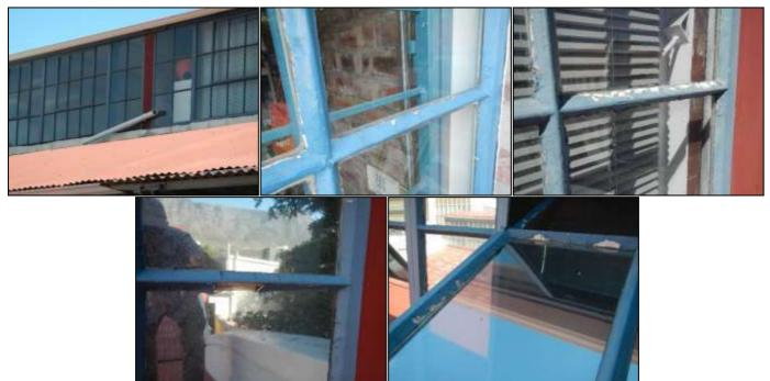
In pictures 1-5 failure of and mechanical damage to the existing metalwork coating was evident in areas.
